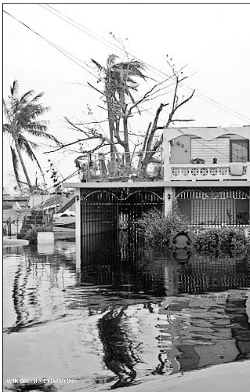
Flooding in Puerto Rico from the Hurricane last year.
